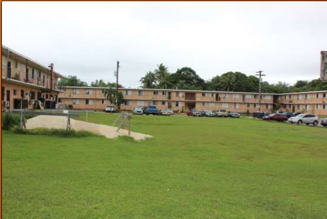
Premier Apartments - October 2017 $5.5 Million ($58,511 per unit of 94 units)
